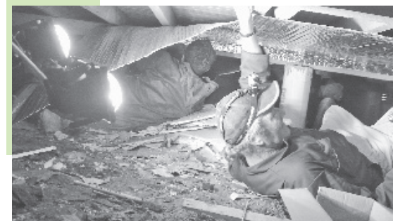
Protection from cold – Karl Hart de Boer fitting underfloor insulation.
