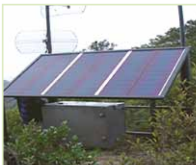
The Tawhiuau Tower site, one of the most remote in the Tūhoe region, is a three hour trek from the bottom of the mountain. Many of Tūhoe Online’s WIFI towers are powered by solar panels and wind turbines.
